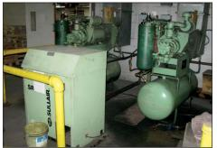
VIEW OF SULLAIR ROTARY SCREW AIR COMPRESSORS
