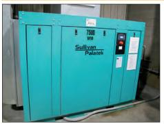
SULLIVAN PALATEK 75 HP ROTARY SCREW AIR COMPRESSOR MODEL 75UD-VFD
