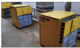
(3) KAESER ROTARY SCREW AIR COMPRESSORS MODEL SK26
