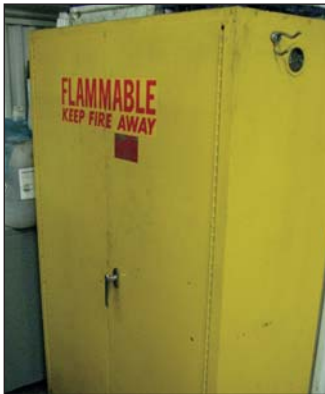
FLAMMABLE LIQUID STORAGE CABINET
