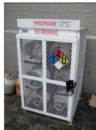
PROPANE SAFETY CAGE
