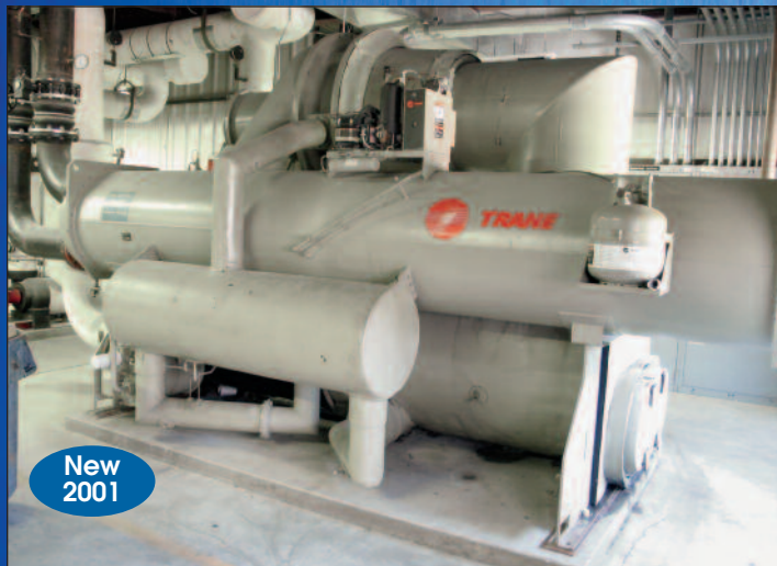
Trane 650-Ton CentraVac Chiller Model CVHF-650
