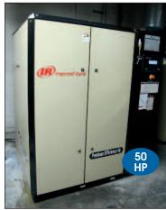
Ingersoll Rand Premium Efficient Air Rotary Screw Air Compressor Model IRN50H-CC
