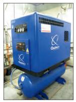
QUINCY 25 HP ROTARY SCREW AIR COMPRESSOR MODEL QGB-25
